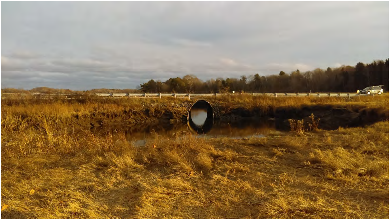
Existing Aluminum Culvert Crossing at Sawyer Road (Photo Credit: Wells National Estuarine Research Reserve)
