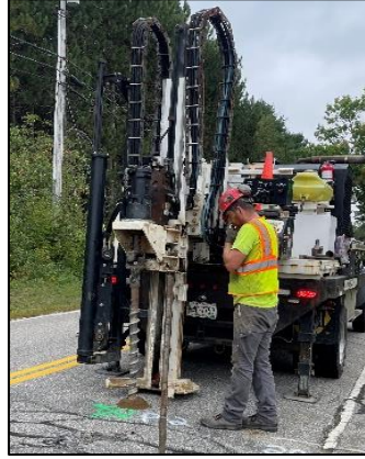
Roadway Borings & Ledge Probes on Mitchell Hill Road
